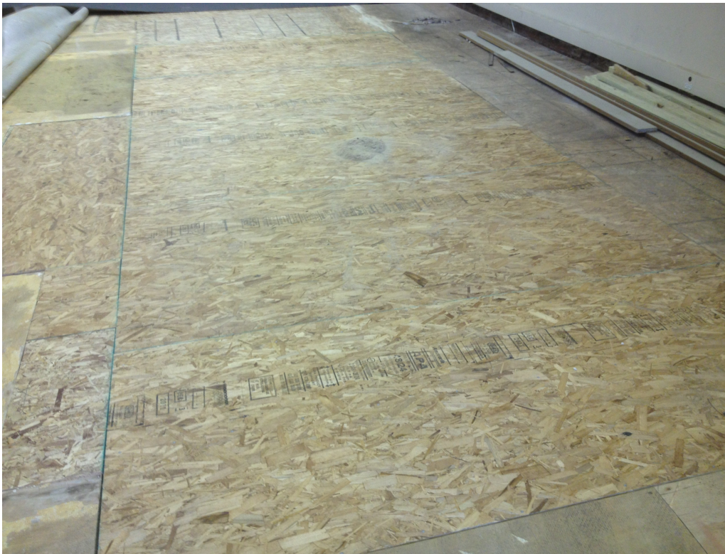
The hole is filled
